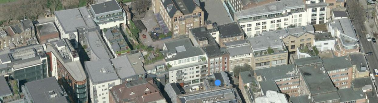
Image 1: Aerial view of street elevation
